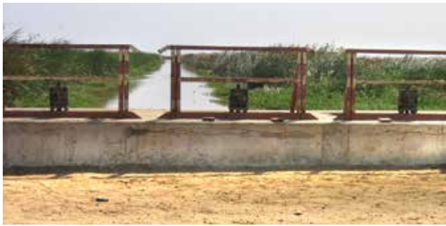
Diawling National Park, Mauritania: The Lemur sluiceway allows flooding of the Bell basin by the Senegal River and was installed as part of a project to restore seasonal flooding to the delta. (Case study 6) © Diawling National Park, Mauritania
