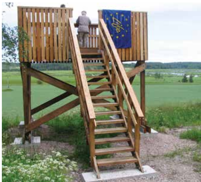
Bird towers are a central element in managing recreational access and visitor experience in restored wetlands. © Viliina Evokari
