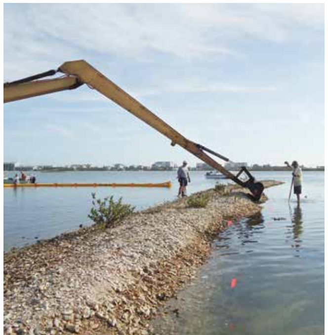
Excavator, Mosquito Lagoon: The overall project goal is to increase the areal coverage of live intertidal oyster reefs by leveling the dead margins and covering the shell material with oyster mats, a stabilized recruitment substrate for oysters. © Anne P. Birch, The Nature Conservancy
