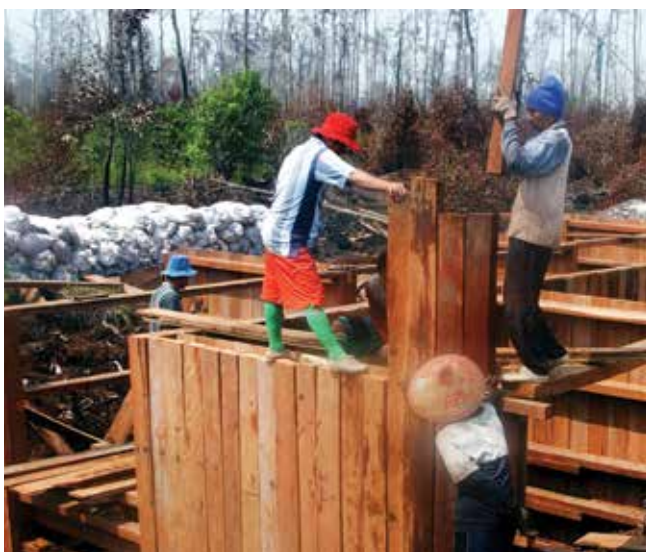
Sebangau National Park, Central Kalimantan, Indonesia: WWF built a canal dam to increase the water level and soil humidity in peat areas. © WWF-Indonesia/Hendry
